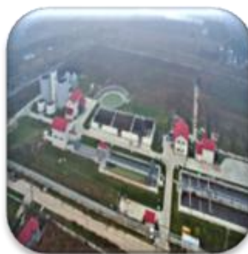
Fig. 1. Călărași Treatment Station Source of data: Călărași Treatment Station.
